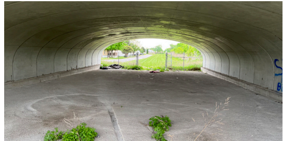
Lincoln Hwy / US Route 30 underpass looking east
