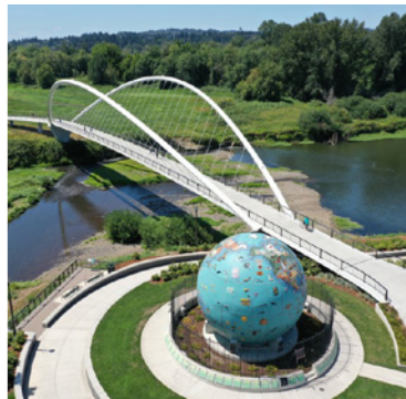
Bike and pedestrian bridge
