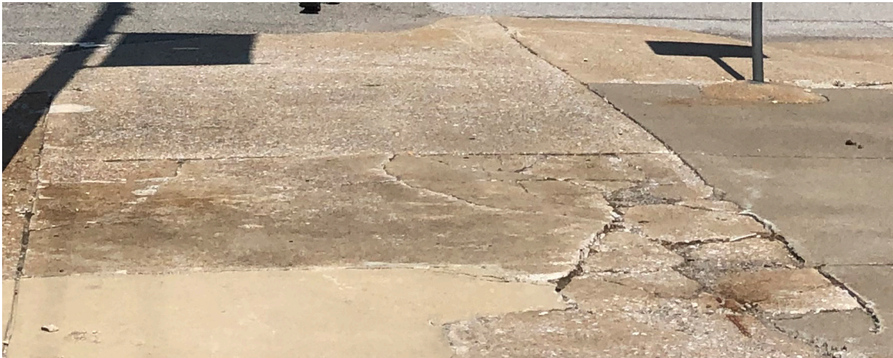
Sidewalk in fair condition on an arterial.
