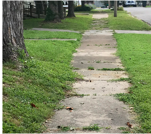
Sidewalk in fair condition on a local street.
